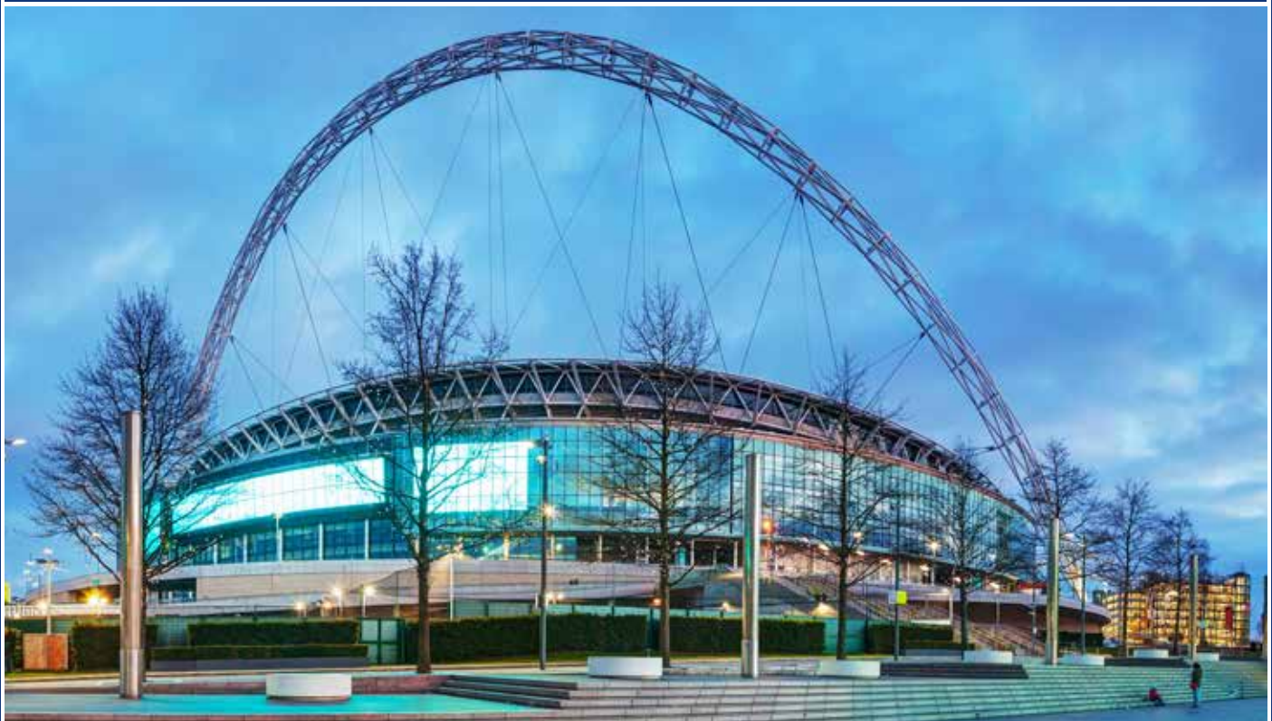
Below Wembley Stadium
